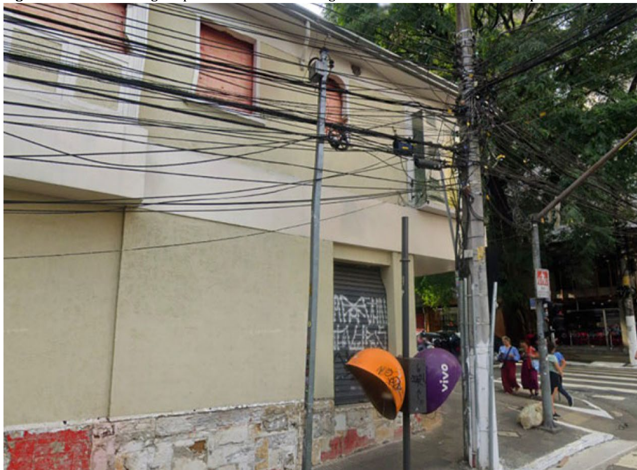
Figure 8 - Photo showing the precariousness and danger of the electric-but-functional poles in São Paulo.
